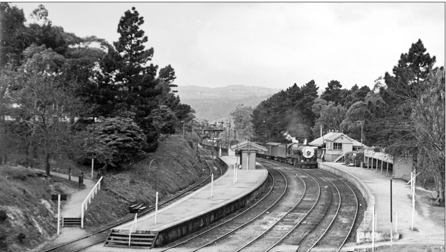
Below. This 1951 photo shows Belair station in about its final form, showing the stone island Down platform, the middle Through Main and, on the Up platform, the stone station building, the signal cabin, the hedge which was planted where the old ticket office was and the platform shelter, now devoid of the enclosed ladies waiting room. A paleface 500 class Mountain Type is coming through on the Up Main on a freight train. Photo: SLSA B 58892/21.
