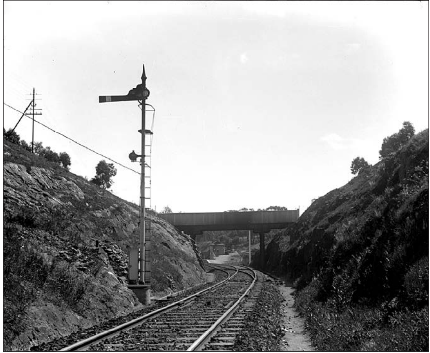
Above. The automatic electric upper quadrant Home signal at the Adelaide end of Belair, introduced in 1924, before duplication reached there in 1928. It governed the entrance to Belair yard through the Down Through Main and the back siding. The Upper Sturt Road overbridge is seen. Photo: Ron Stewien, NRM Archives.
